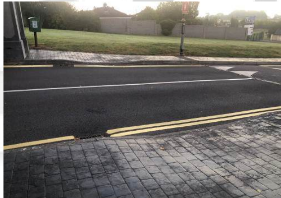
Photograph 6: Kingsfort Avenue Adjacent to St. Joseph's Road Junction
