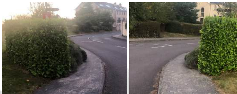
Photographs 3-4 : Kingsfort Avenue Footway & Sign Restricted by Vegetation
