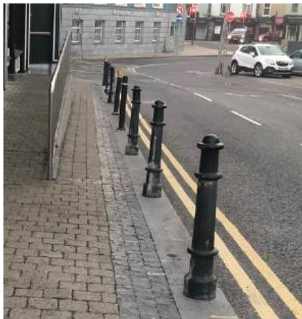
Photograph 11: View South West of St. Joseph's Road North West Side Footway
