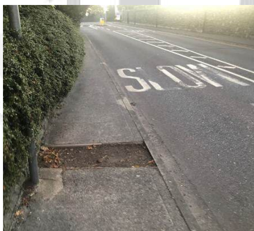
Photograph 8: View North East of St. Joseph's Road North West Side Footway
