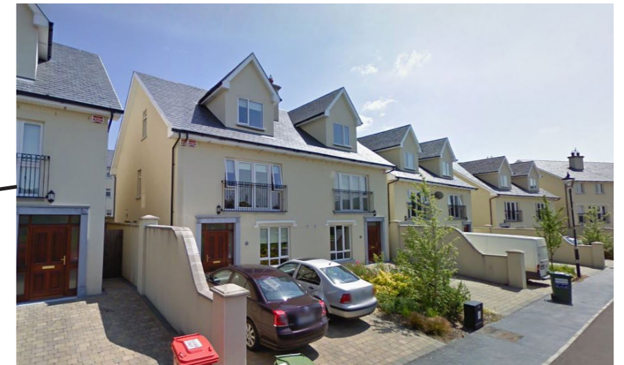
2.5 STOREY UNITS ON MAPLE AVE
