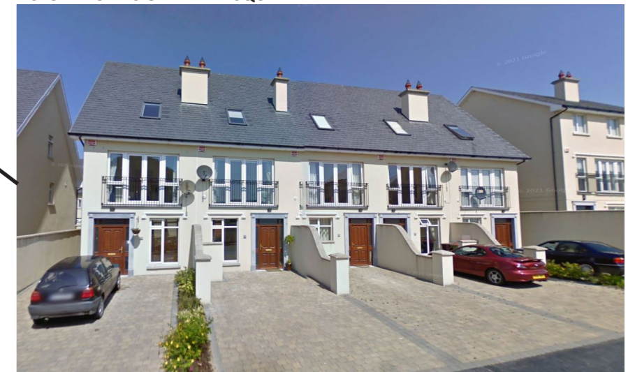
2 STOREY UNITS ON MAPLE SQUARE
